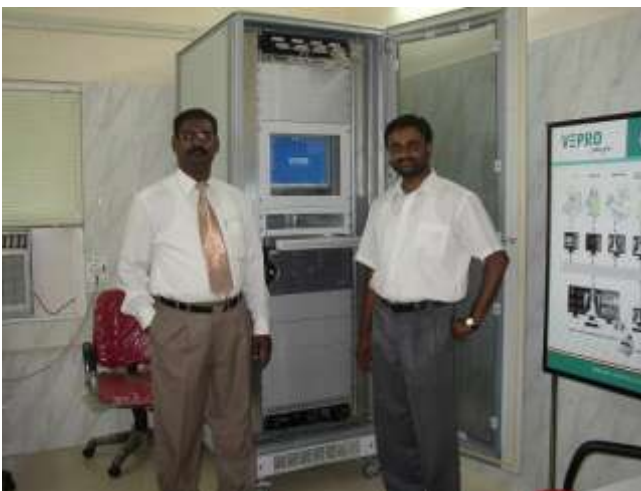
Main Archive Server rack
